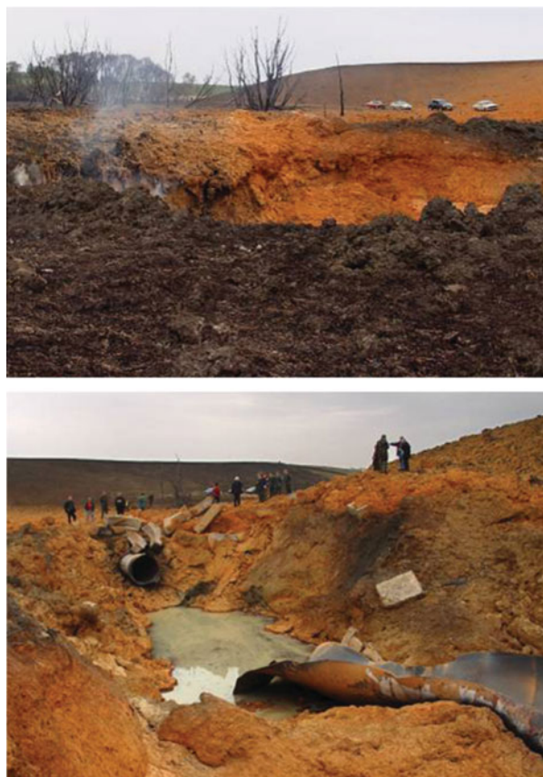
Fig. 1. The results of the Urengoy–Pomary–Uzhgorod pipeline disaster for the environment
