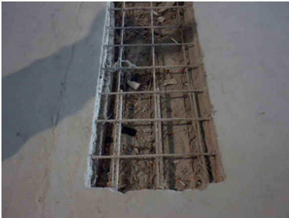
Fig. 3. View of the spatial trusses of composite deck slab
