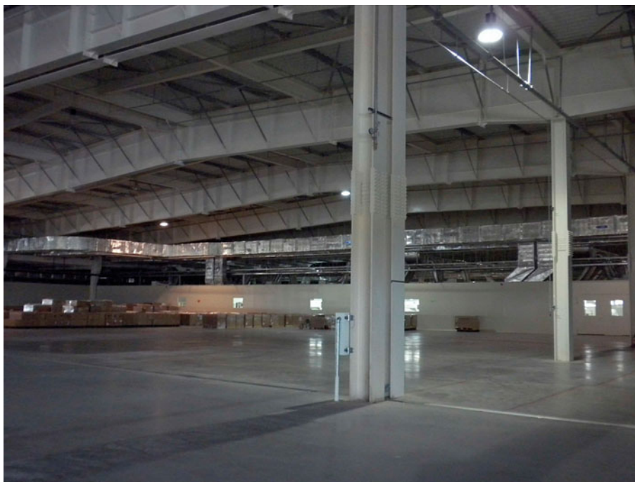
Fig. 1. General view of steel-bearing structure of the industrial hall
