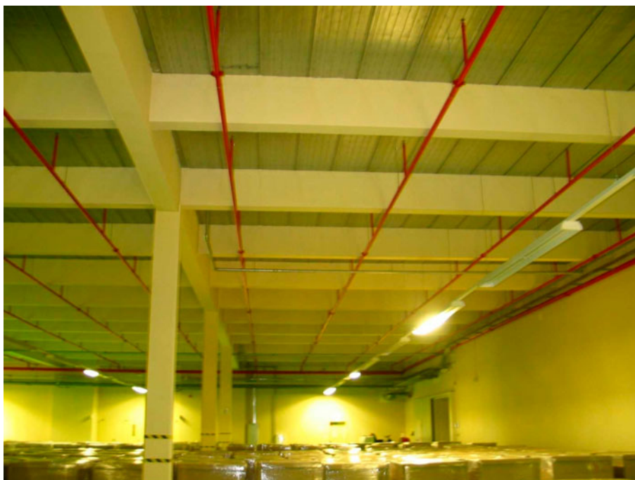
Fig. 2. View of the system of main and secondary floor beams
