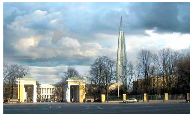
Fig. 5. Okhta Centre (known until March 2017 as Gazprom City) would ruin the city's appearance
