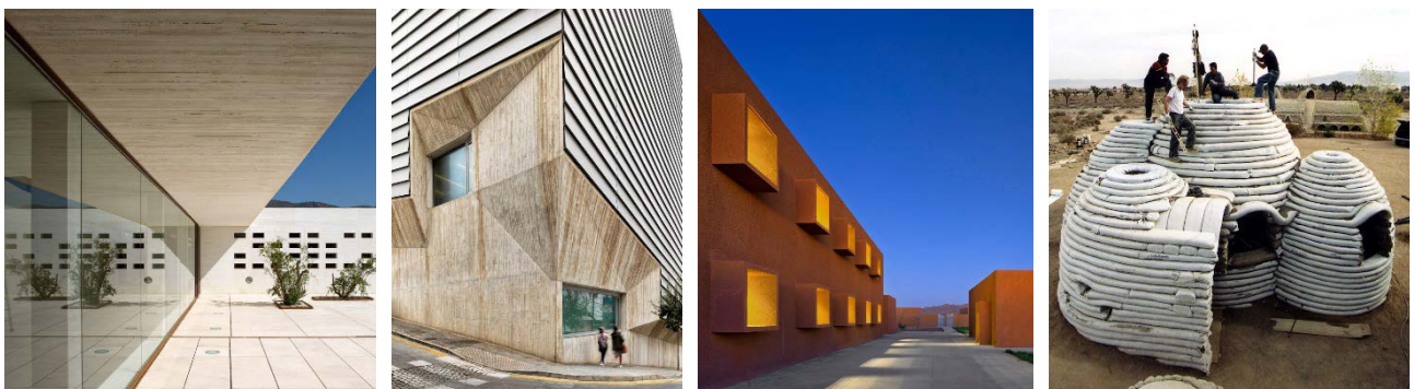
Figure 4. Madinat Al-Zahra Museum (Córdoba, Spain); Ceuta Public Library (Ceuta, Spain); Guelmim School of Technology (Guelmim, Morocco); Sandbag Shelter Prototypes (Ahwaz, Iran) (right to left)
